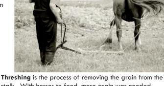
Threshing is the process of removing the grain from the stalk. With horses to feed, more grain was needed. The early threshing machines were horse powered with the stalks hand fed. From the late 1800's steam powered machines became more available and rapidly replaced this once very laborious task.
